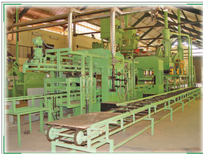
PARTICLE BOARD PLANT
